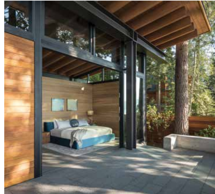
THIS PAGE CLOCKWISE FROM TOP: The built-up roof was constructed using clear span re-sawn rafters that are sitting on heavy gauge steel I-beams spanning 91 feet. Installed by Vertical Iron Works, the steel structure supports the roof load and allows the large sliding glass door opening | The primary suite has its own 15-foot-wide sliding glass wall that allows easy access the lakeside patio | The 10-foot-tall entry pivot door served as the datum point of the entire house—where the exterior walkway leading from the garage to the home precisely lines up to the center of the great room and lakeside patio doors OPPOSITE PAGE FROM TOP: The office has custom scraped walnut floors along with T&G knotty cedar ceilings to provide the room with some warmth | Bentwood walnut cabinetry with integrated matte black pulls by Truckee Tahoe Lumber Design Center create clean horizontal lines
