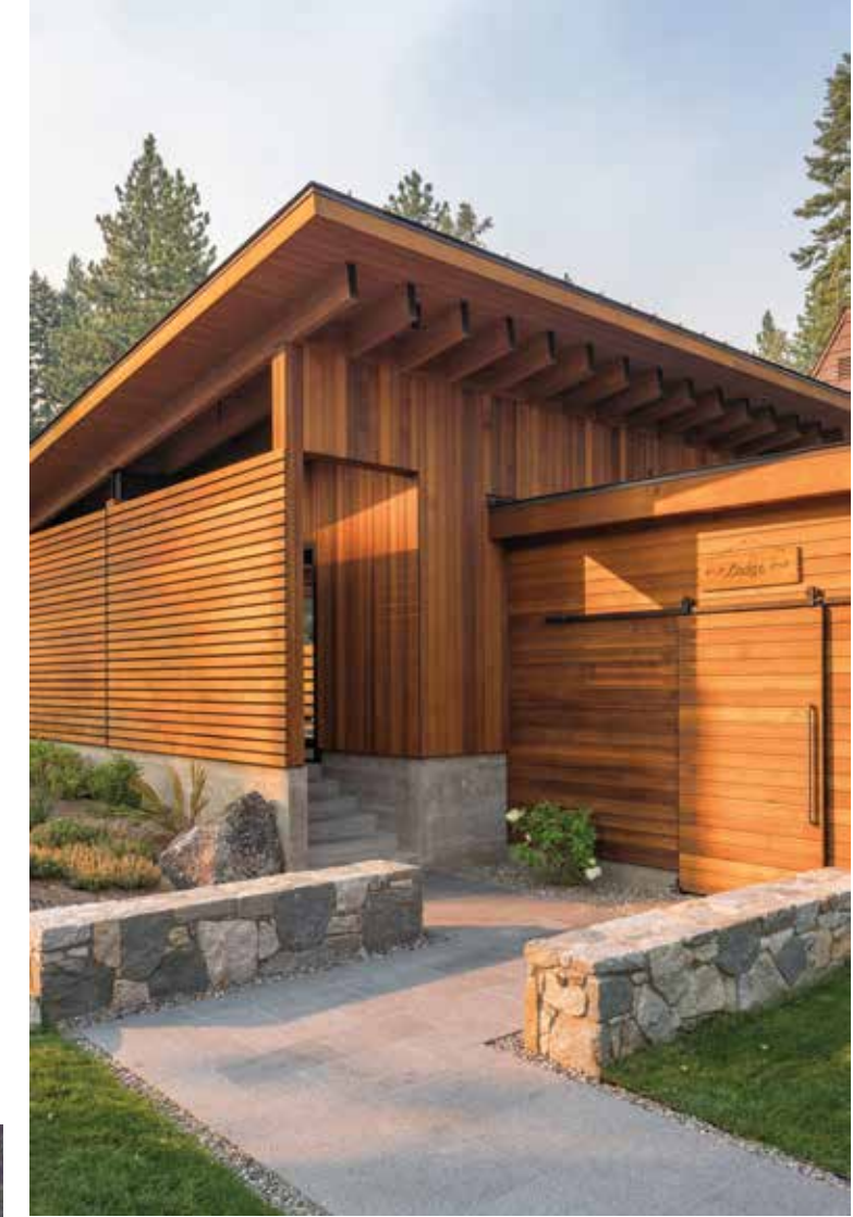
FROM TOP: Alongside the detached garage, horizontal custom-milled cedar boards with 3/4-inch spacing were used as an open-air privacy wall that delineates the entry breezeway and exterior courtyard | An elevated view of the 84-foot-wide home from the shoreline of Lake Tahoe showcases the expansive glass walls and interior finishes
